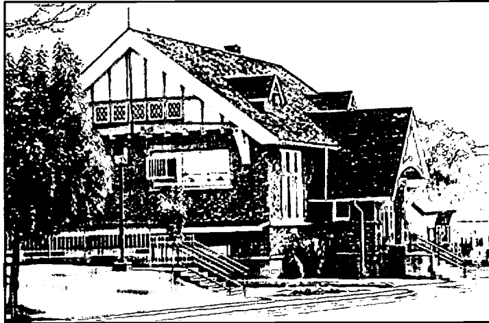
(Richfield Public Library, Richfield, Utah)
