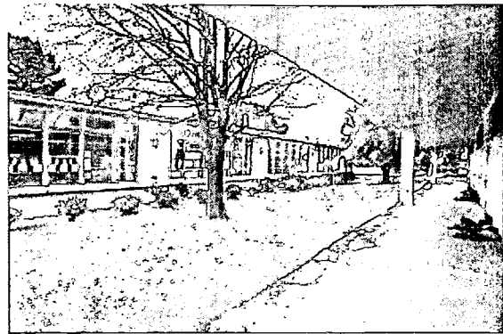
North versus south windows-south windows are shaded from direct sun-but receive daylight reflected off of concrete walk and white painted overhangs. North windows are large and unshaded.
