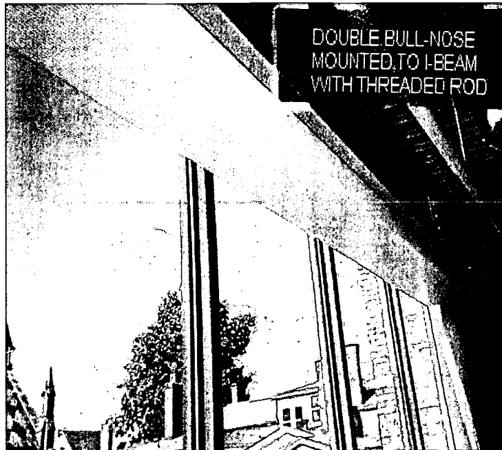
Extruded Aluminum Linear Panel. NREL/PIX 11422
