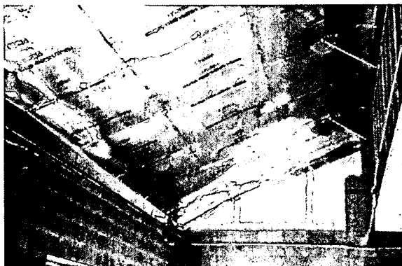
Radiant barriers are recommended for hot and coastal climates, over spaces cooled by air conditioners or natural ventilation. NREL/PIX 11331
