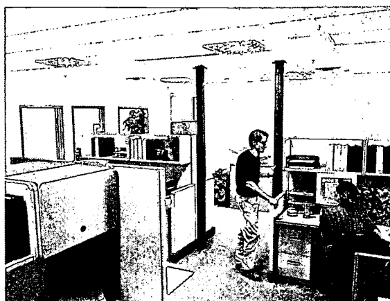
Tubular skylights in interior administrative office provide high lighting levels even when electric lights are off. Skylight diffuser panel fits into a standard suspended ceiling system.
