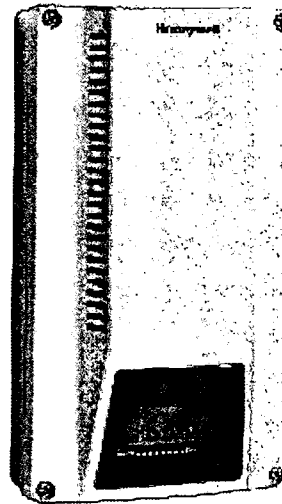
CO 2 sensors help indicate building occupancy levels, allowing for better control of the quantity of ventilation air needed. NREL/PIX 11425
