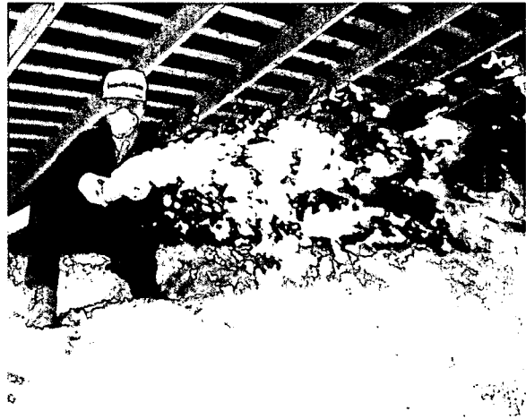
Well-insulated roofs and roof cavities can reduce drafts and thermal loads in buildings. NREL/PIX 11421
