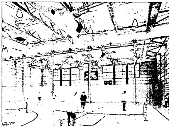
Metal halide luminaires are one option for general lighting in gymnasiums. NREL/PIX 11437
