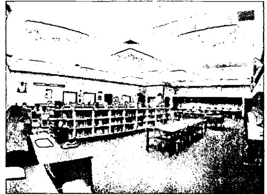
Deeply coffered ceiling helps to diffuse light from four skylights. There are no electric lights on in this photo. NREL/PIX 11470
