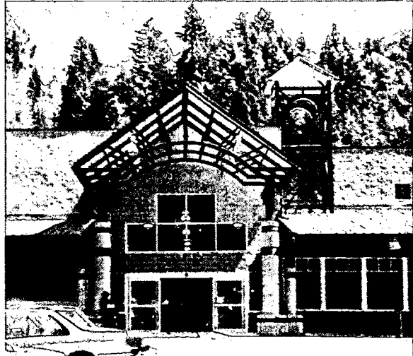
The concrete masonry unit used at this market had considerably lower first costs than would traditional, framed walls. NREL/PIX 11412
