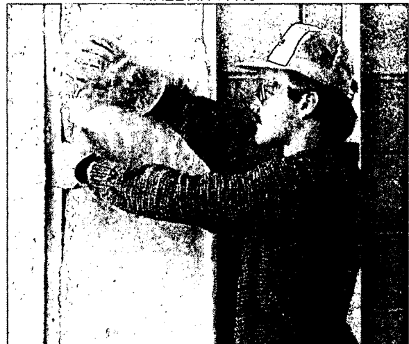
Masonry walls can be insulated on the interior, but the benefits of thermal mass are mostly lost.
