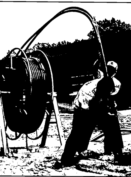
Photo: Advanced Energy
