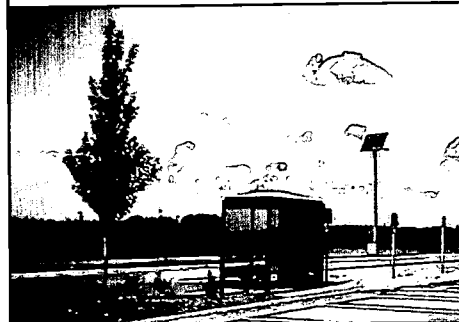
These stand-alone photovoltaic systems power parking lights.
