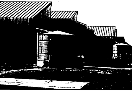
Roy Lee Walker Elementary School, in McKinney, TX, collects 700,000 gallons of rainwater each year.
