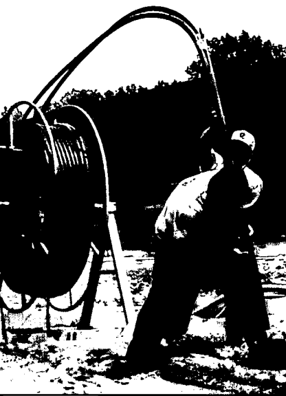
Photo: Advanced Energy
