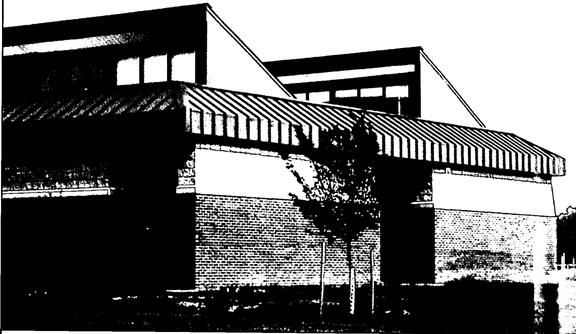
Clear glass for south-facing roof monitors and low-e glass for view windows are two daylighting and energy-efficient features.
