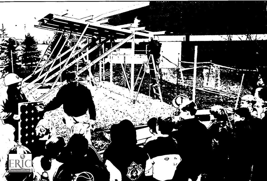
Photo: Bluffsview Middle School Photovoltaic systems can be great teaching tools as well as energy savers.
