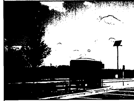
These stand-alone photovoltaic systems power parking lights.
