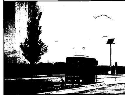
These stand-alone photovoltaic systems power parking lights.
