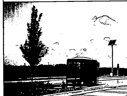
These stand-alone photovoltaic systems power parking lights.
