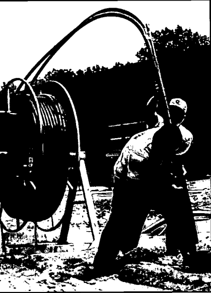
Photo: Advanced Energy
