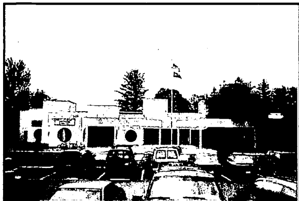
Figure 2.14: Sweetbriar Elementary School, Troutdale
