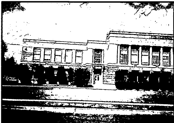
Figure 2.4: Evergreen Elementary School, Redmond
