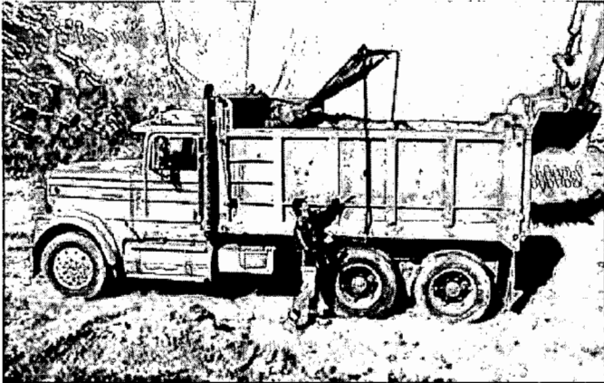
Excavation equipment working on the construction site.
