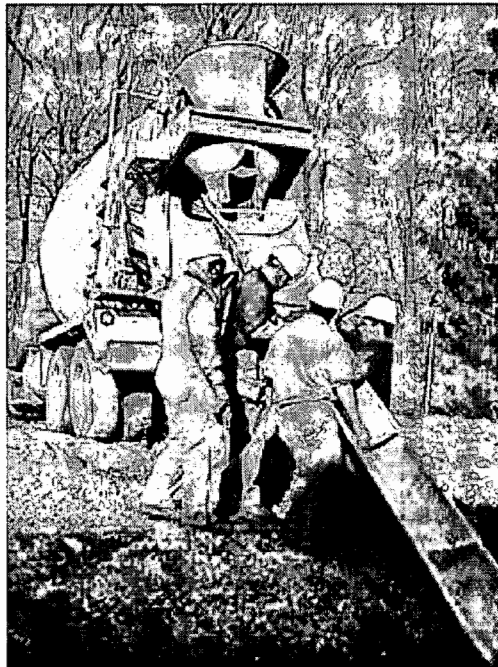
The concrete trucks arrived and began to pour.
