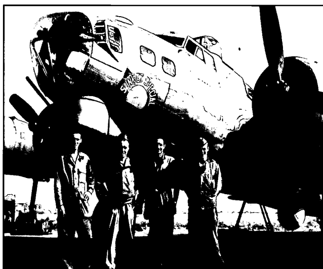
PATHFINDER MAINTENANCE CREW (NOTE RADAR DOME REPLACING BALL TURRET GUNS)
