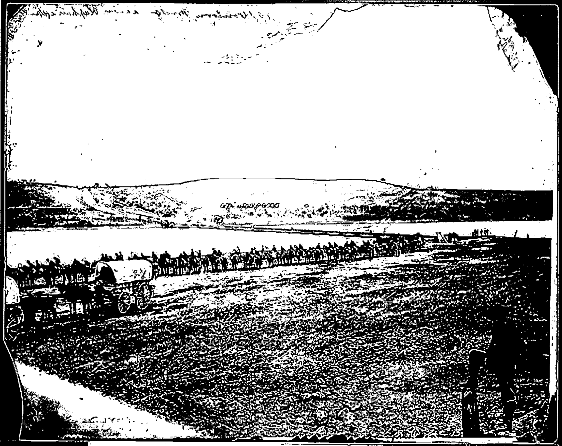
Document 4: Pontoon across the Rappahannock River, Virginia, Cavalry column
