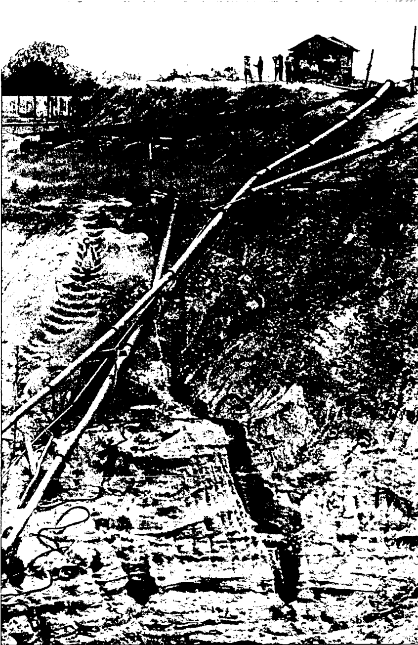
The soil and water are pumped up the hill.
