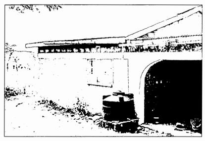
We collect rainwater in this black tank (400 litres) from our roof. During the rains the water over flows, so we frequently empty it into other buckets.
