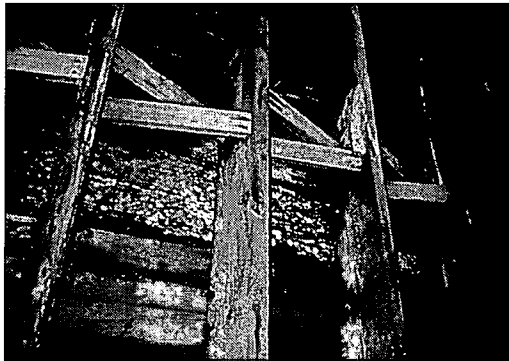
Photo 6: Heavy mold growth on underside of spruce floorboards
