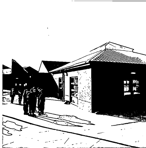
Figure 5/4 The new extension at Standish School.
