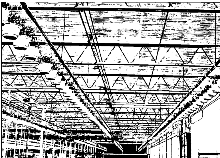
Figure 3.21 Interior ceiling at eave height
