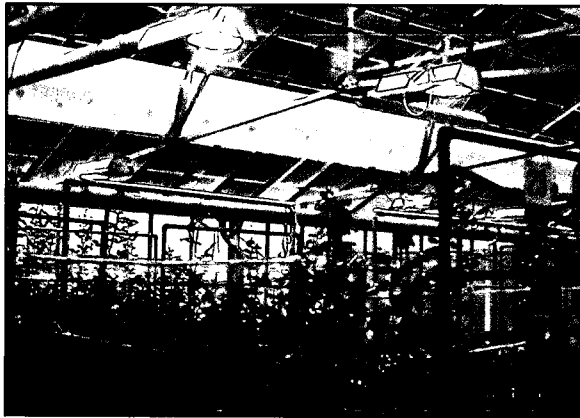
Figure 4.17 High Intensity Discharge (HID) 400-watt lamps in operation.
