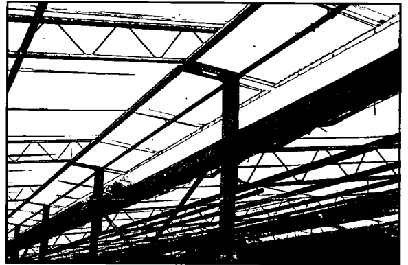
Figure 3.49 Fiberglass ridge vent that is open. When the pipe rotates 90°, the vent will be closed.
