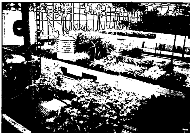
Figure 3.6 Temperature sensor suspended just above a bench. Note white fins through which air is drawn by a fan at the bottom of sensor housing.
