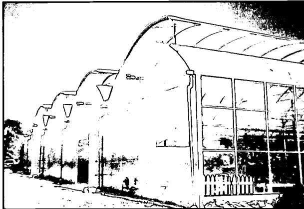
Figure 3.55 Exterior view of a barrel vault ridge-and-furrow greenhouse range with roof vents open.
