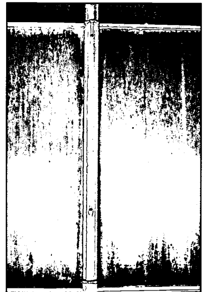
Figure 2.16 Close-up view of an aluminum sash bar showing the sash bar cap
