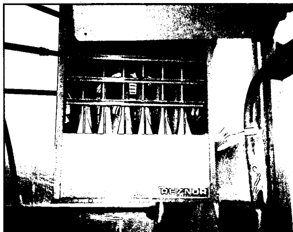
Figure 3.11 Front and back views of a gas-fired horizontal unit
