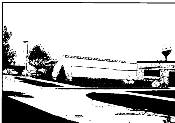
Figure 3.44 Whitewash applied to the outside of a greenhouse
