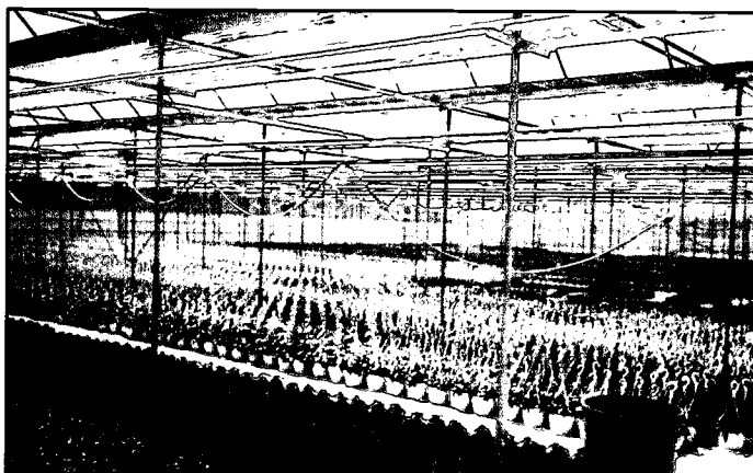
Figure 5.30 A shade curtain drawn across the greenhouse lowers light intensity.
