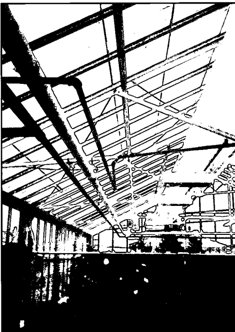
Figure 2.11 Typical even-span construction showing a purlin running the length of the greenhouse, supporting the sash bars and connecting the trusses
