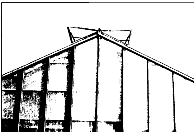
Figure 3.27 Open ridge vents in a greenhouse. Note white shading compound sprayed on the end wall.
