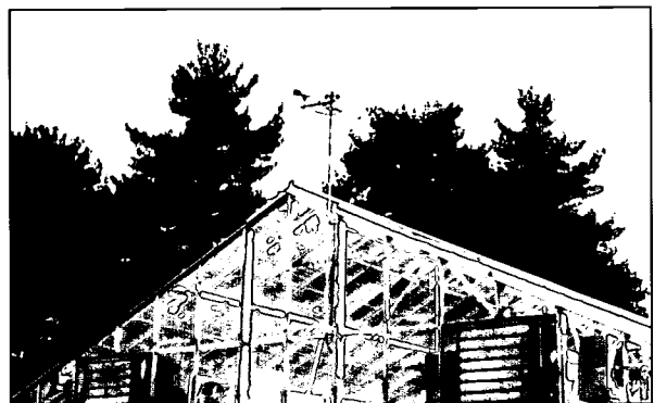
Figure 5.29 Weather station installed on greenhouse roof.
