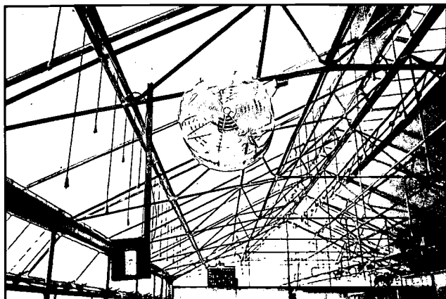
Figure 3.20 Horizontal air flow fan mounted from a chord at eave height. Fans in the other half of the greenhouse are facing the opposite direction.
