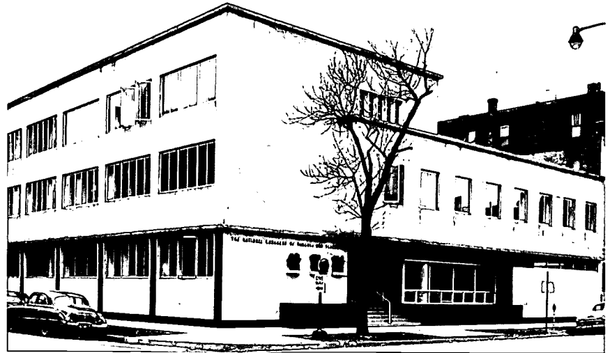
The building at 700 N. Rush Street was home to the National PTA until November 1993, when the PTA moved its headquarters to the IBM Building in Chicago. Prominent features of the building's entrance were three bronze statues (below, left) created by Chicago sculptor Milton Horn. The statues symbolize the Mother, the Father, and the Teacher as the most important influences in children's lives.
