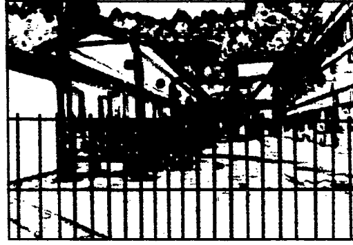
Wrought-iron fencing reestablishes access control without compromising natural surveillance.
