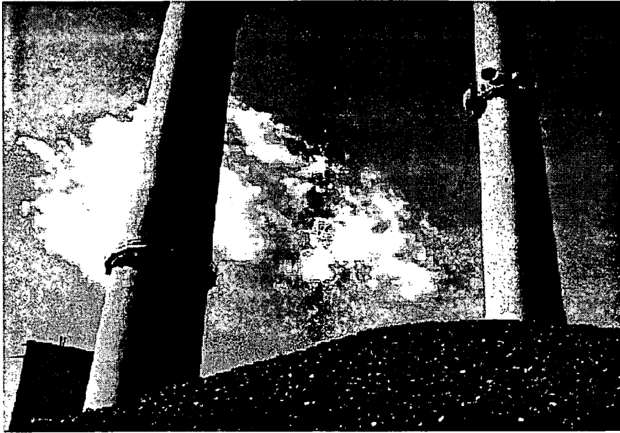
This Union Electric Power Plant uses scrap tire chips as part of its fuel, replacing a portion of coal burned.
