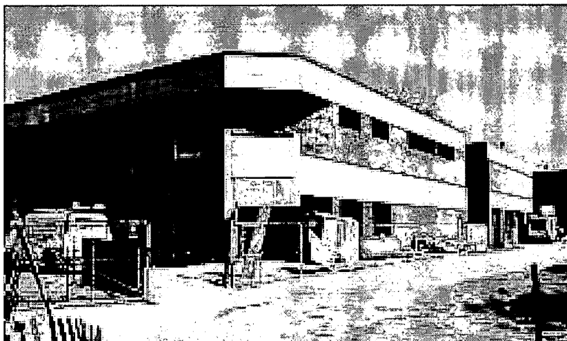
This is a picture of the Health Building under construction.
