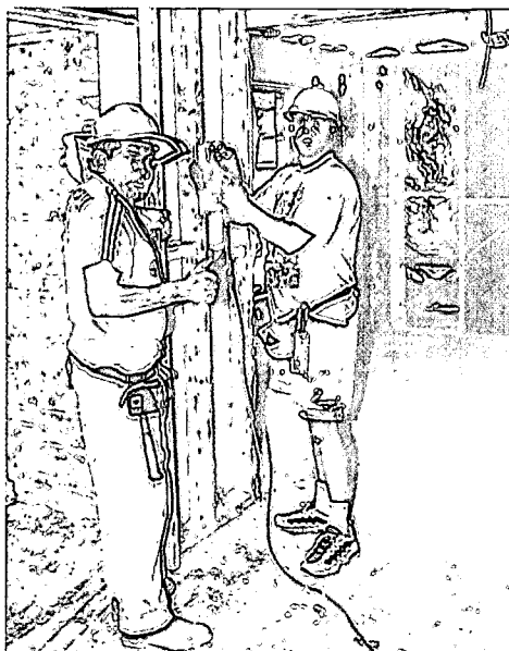
Carpentry students at Western Institute's Dubbo Campus, TAFE NSW, building community housing for Aboriginals.
