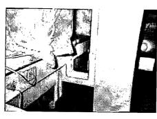
The communications wiring would be placed by the state contractor so one channel was reserved for that application. Tony and his assistants placed the electrical wiring into one of the other channels. Standard single-gang electrical outlet boxes were placed every few feet. Later on, when the state contractor placed the communications wiring, all they had to do was remove the cover, place the cable and set the boxes for modem devices right into the raceway. It went without a hitch
