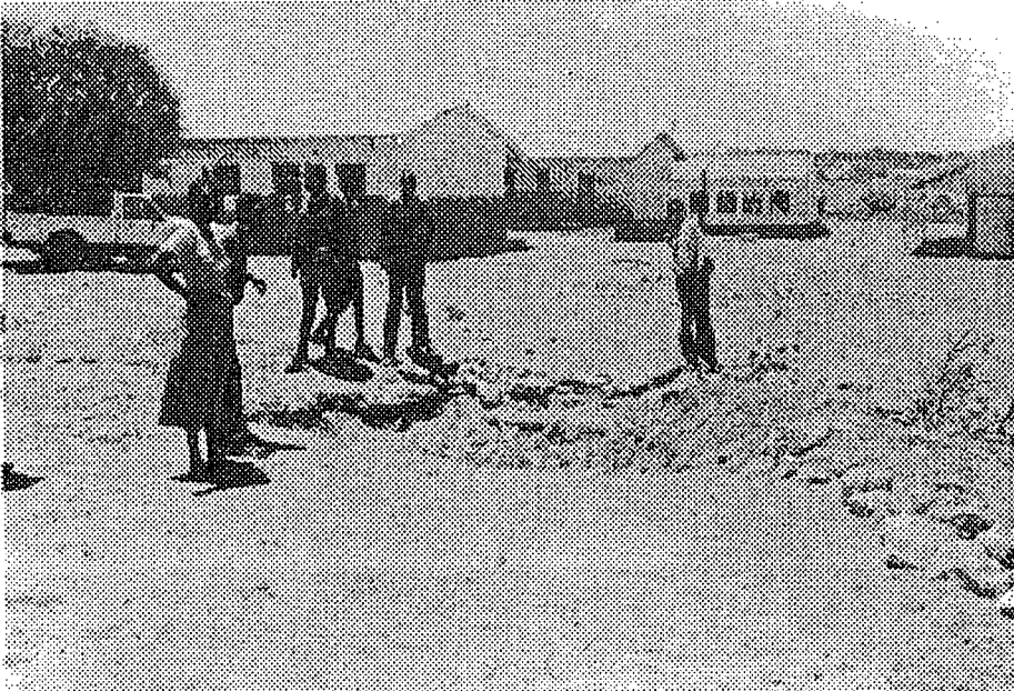
Figure 1: The pit of a micro-catchment that harvests run-off rain water from the school grounds. Most of the water gets trapped in the pit so that it can slowly infiltrate into the surrounding soil. Trees and vines are planted around the pit to make use of this water. Any excess water can escape over the stone spillway at the fence.
