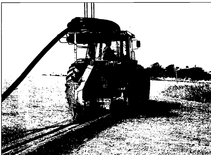
A tractor installs playing field drainage.
