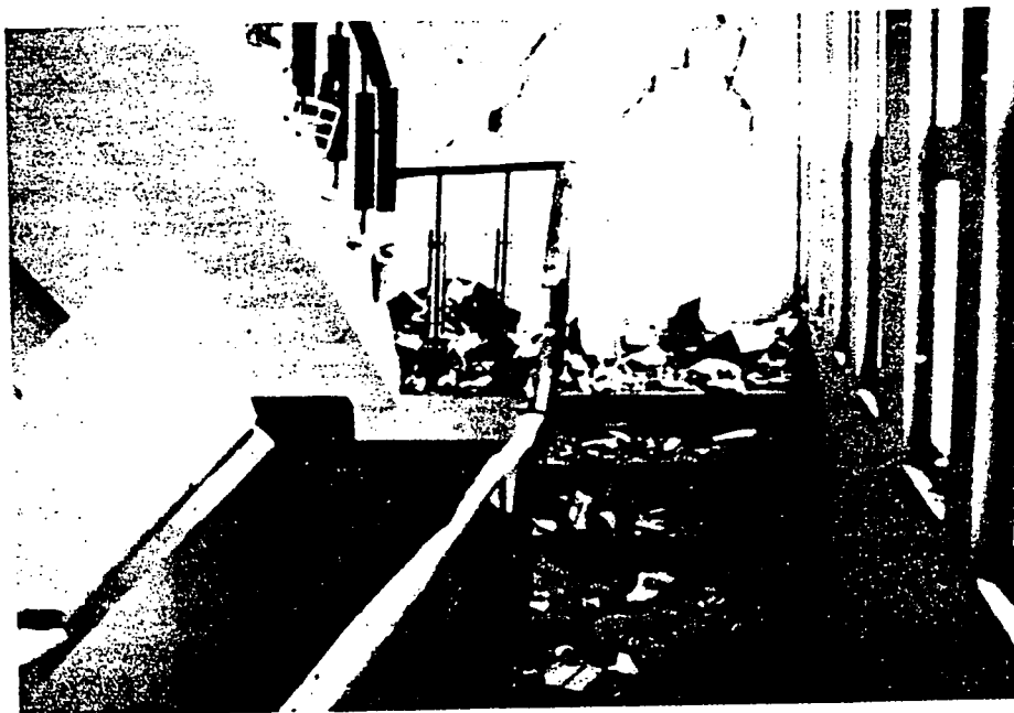
FIGURE 24 Stairway failure.
