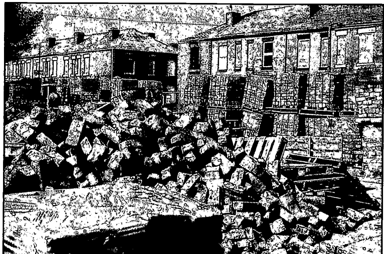
Below: Brick reclamation and recycling [Trevor Perry Environmental Picture Library]
