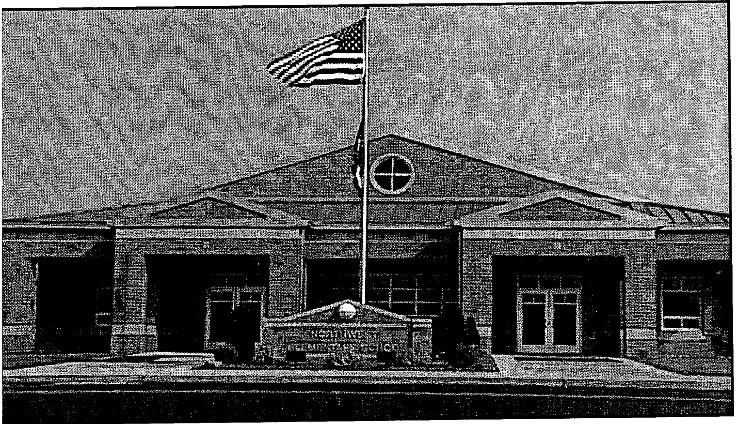
Northwest Elementary School, Scioto County
