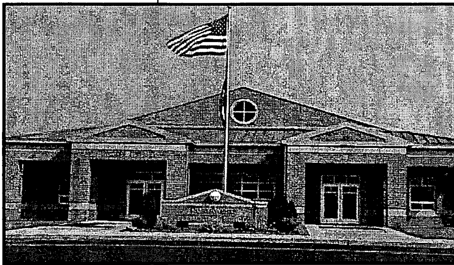
Northwest Elementary School, Scioto County
