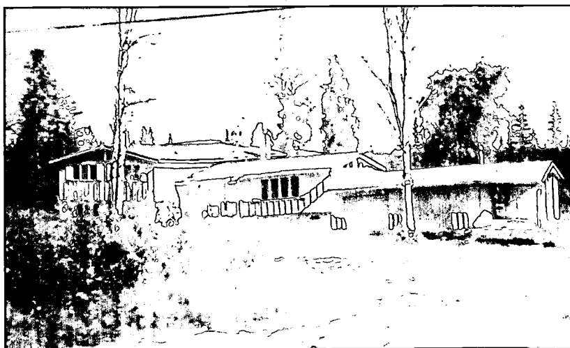
This house was built on ice-rich permafrost. Heat from the house caused the permafrost to thaw and the ground surface to settle unevenly resulting in bending and twisting of the structure which was ultimately abandoned (photograph by Tom Osterkamp).
