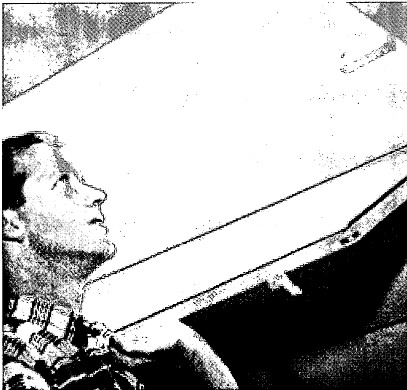
Figure 11. Pasco County School Board Energy Coordinator, Mike Woodall, assists with the time delay adjustment of one of the ceiling mounted occupancy sensors. The project found that proper set-up of the time delay and sensitivity of the controls was essential to acceptable performance.
