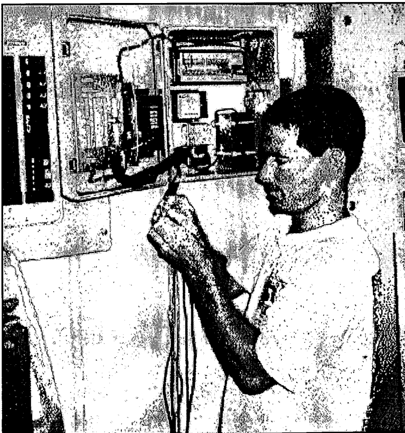
Figure 6. John Sherwin wires in data logger to collect 15-minute data on weather, building thermal conditions, and cooling system electric power.
