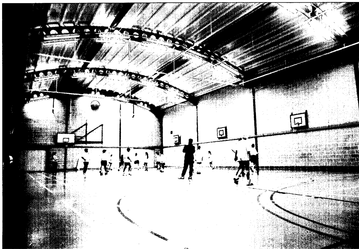
Figure 40: Sports Hall at Oakmead School, Bournemouth, fitted with occupancy controls to switch on lights only in parts of the hall which are in use. - [Photo: Ex-Or Limited]
