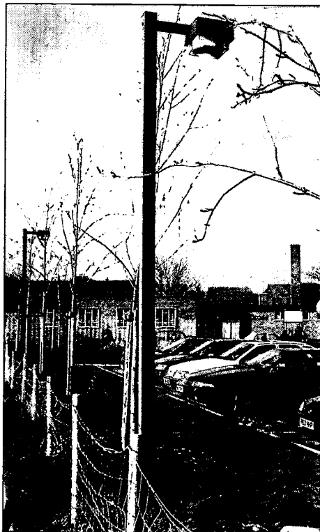
Figure 43: Lighting of footpath with a luminaire which projects light in a downward direction. [Photo: P. Locker]
