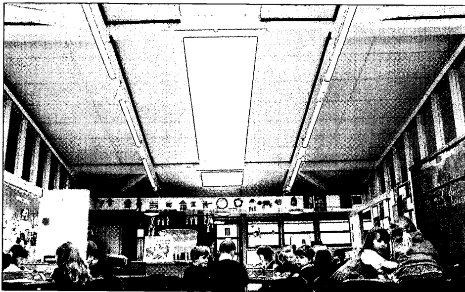
Figure 3: Complementary localised lighting using lines of suspended fluorescent luminaires and display spotlights either side of a central rooflight fitted with louvre blinds (see also Fig. 22). [Photo: P. Locker]
