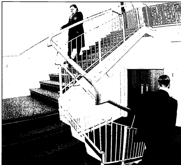
Daylighting of staircase with contrasting treads and risers and avoidance of glare from windows. [Photo: P. Locker]
