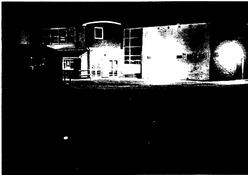
Security Lighting at Hayes Park Primary School (Case study 2).
