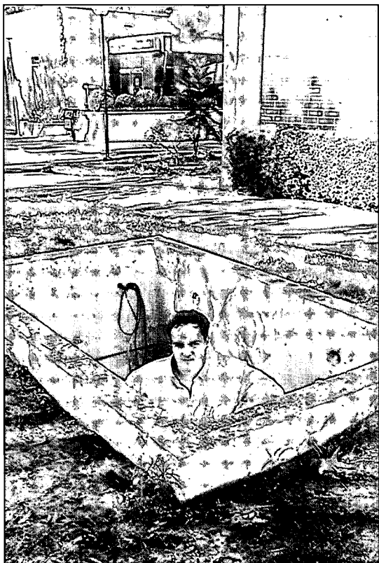
Orange Coast College geology professor, Erik Bender, stands in a new seven-foot-deep earthquake measurement vault on campus. The vault sits atop a 300-foot vertical shaft that contains a sensor at the bottom. The sensor is connected to one of the college's seven seismographs. OCC is the only agency that actively measures earthquakes within the borders of Orange County.
