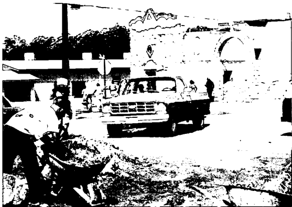
Local Doña Ana youth learn marketable skills in historic building practices at the Neustra Señora de la Candelaria church. Photo by Ed Crocker.
