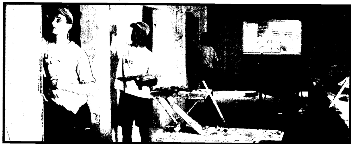
Plastering apprentices at work.
