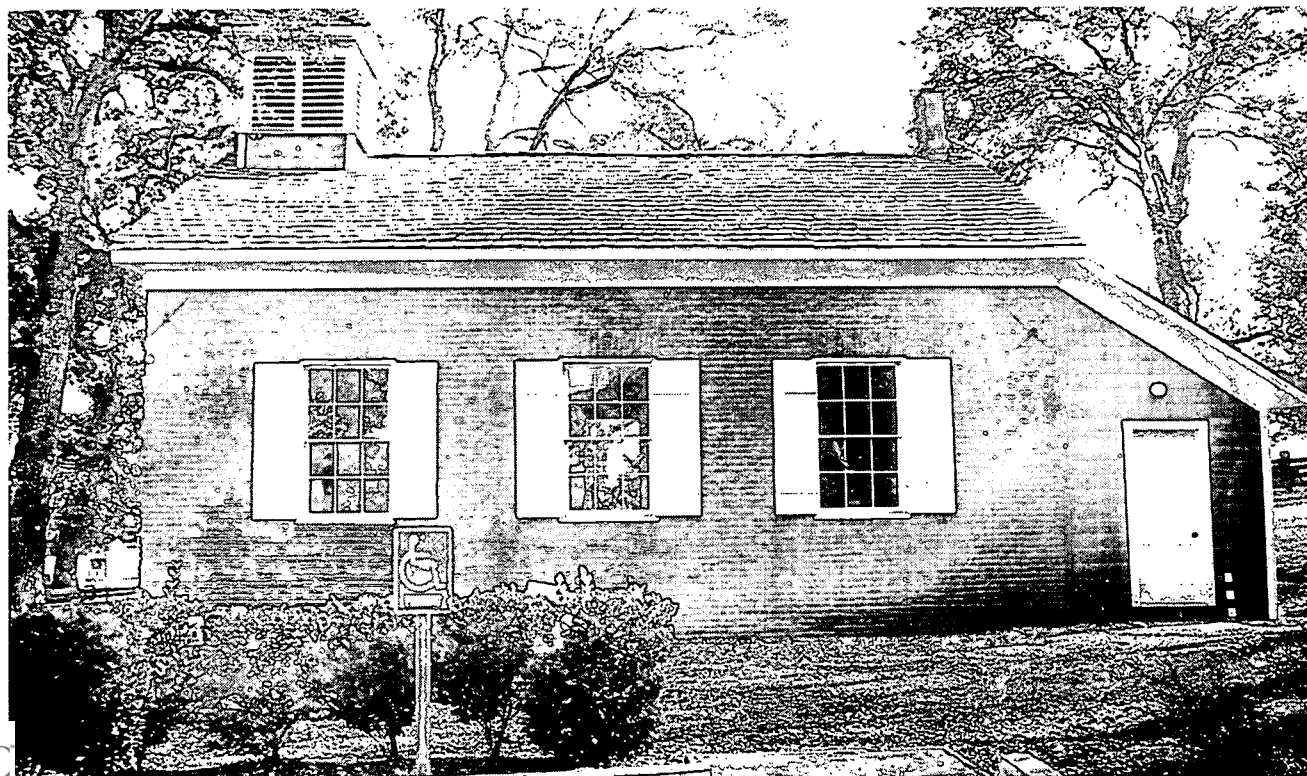
Figure 25: The Altaville School (west elevation) in its present-day renovated condition, serves as a memorial and museum, November 1996. -CSUS/IAR Photo
