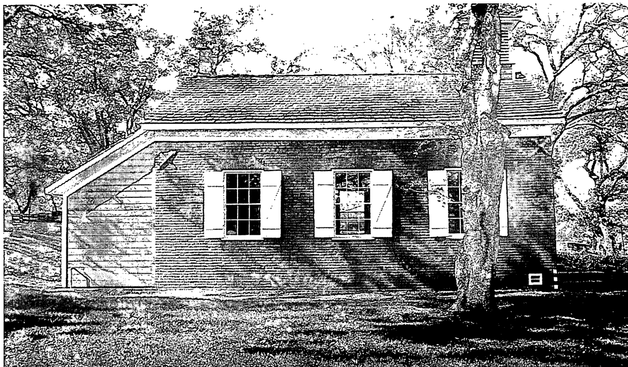
Figure 24: The Altaville School (east elevation) in its present-day renovated condition, serves as a memorial and museum, November 1996. -CSUS/IAR Photo
