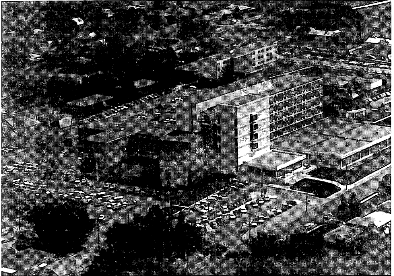
In the 1970s, laboratory facilities, social services, and the front lobby were expanded.
