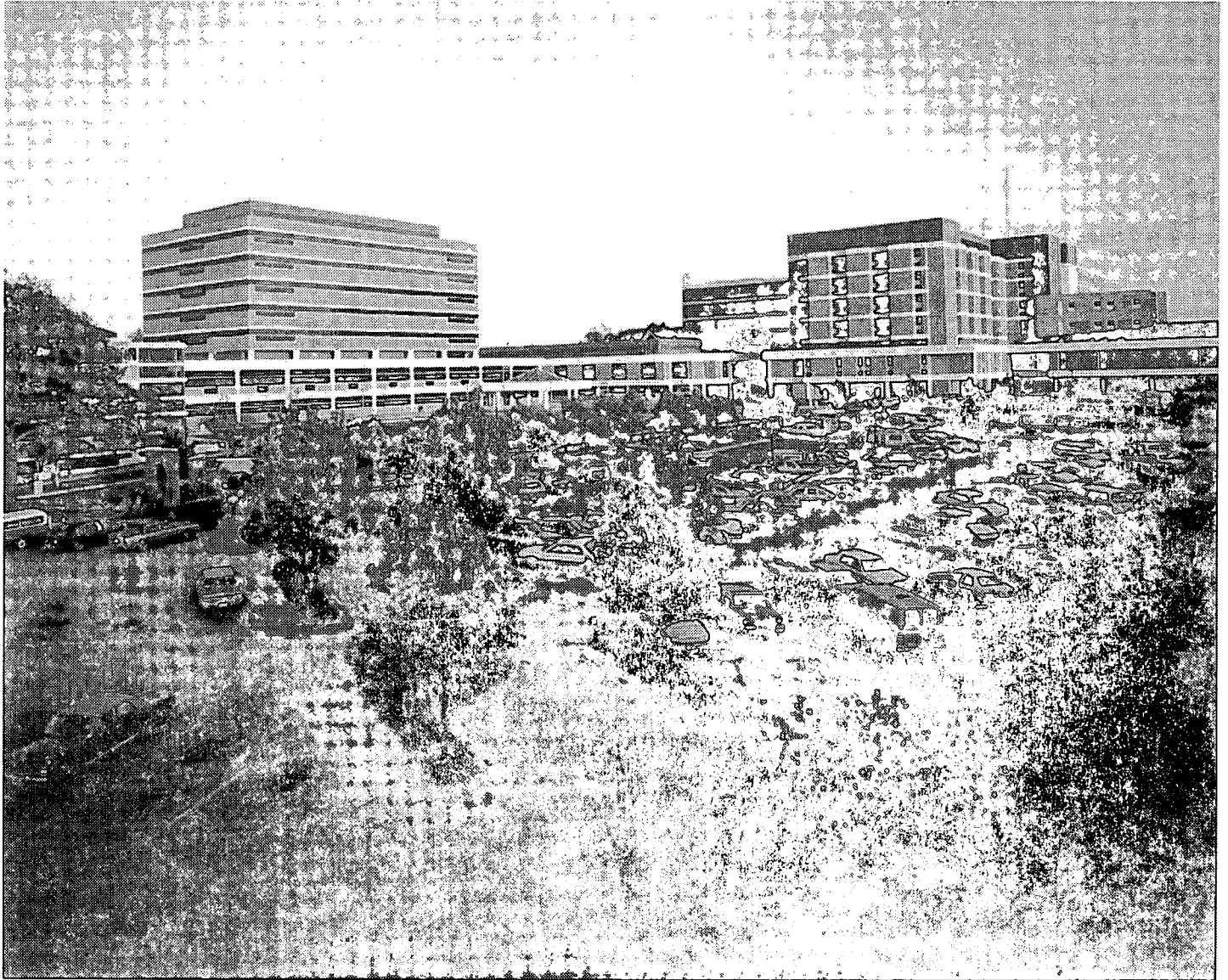
Bryan Memorial Hospital Campus in the 1990s including the outpatient area, the medical office building, and the parking garage.
