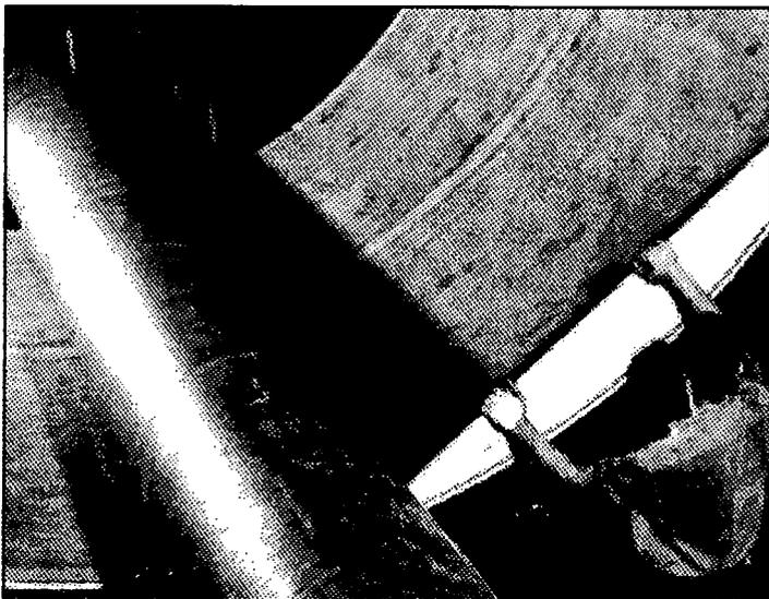
Steel under giant rolls being shaped for submarine construction at the Electric Boat Co., Groton, Conn., in August 1943. (Photo Courtesy National Archives)
