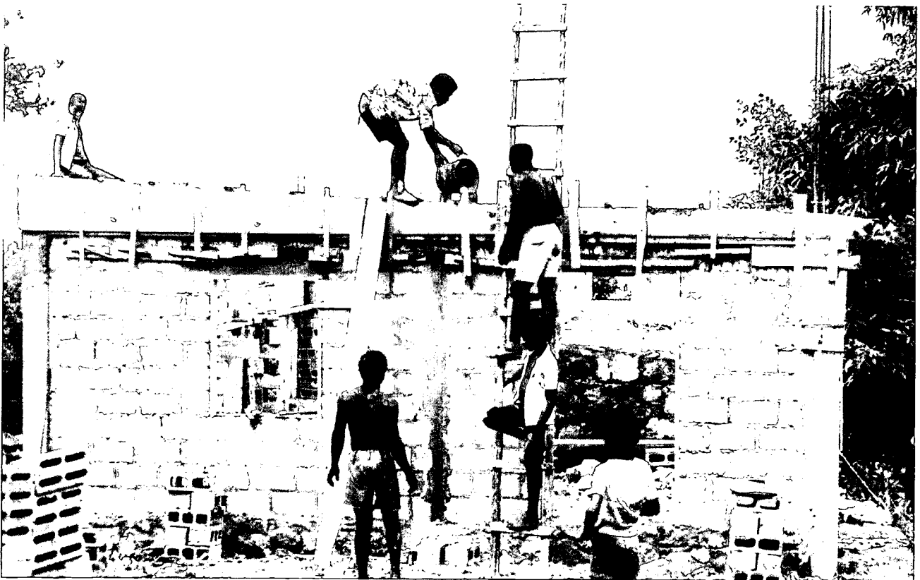
Building a cooperative bakery in Dominica.
