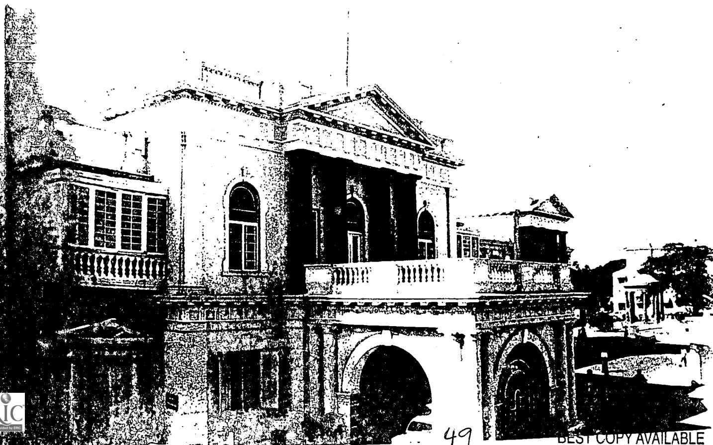
The famous black Doric columns of Pallavaram gneiss once linked Pitt's colonnade with the Sea Gate. In 1910 they were incorporated into the new Council Chamber.
