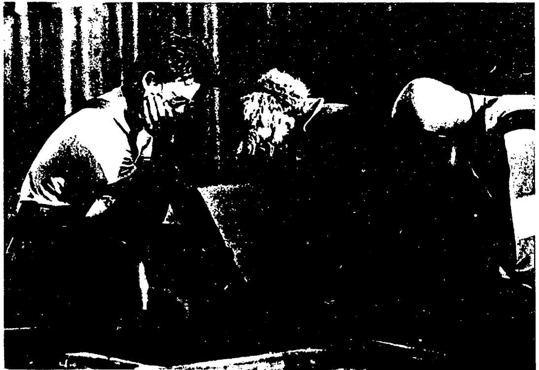
Mark, Nancy, and Mike laying out bay window for House 23 in Construction Technology class
