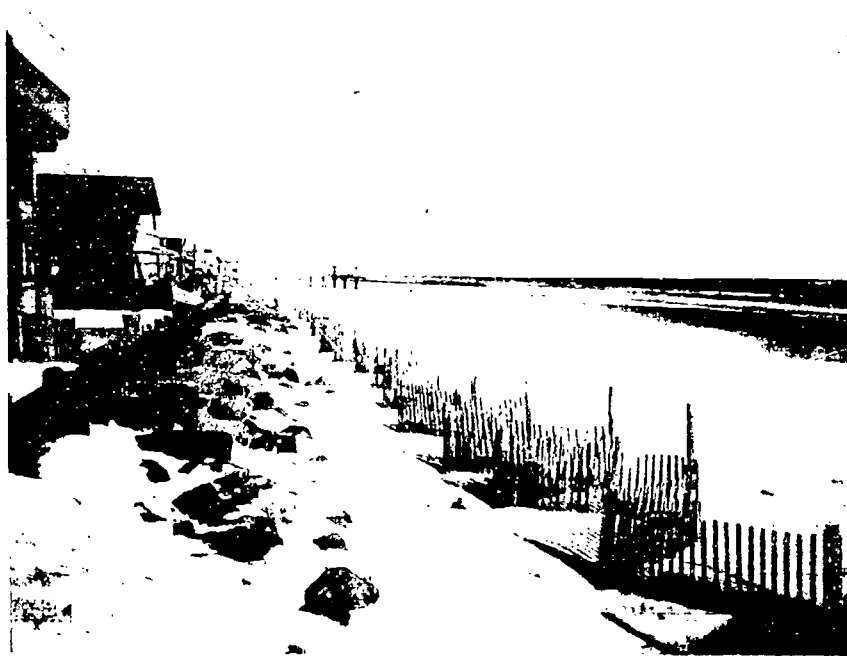
Fig. 6-6. Snow fences, or windbreaker fences, are constructed along beaches to collect airborne sand particles.
