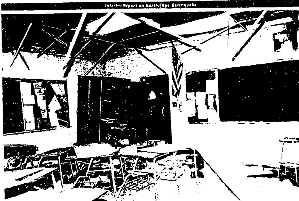
Falling ceiling tiles and light fixtures in classroom at Kennedy High School in Granada Hills
