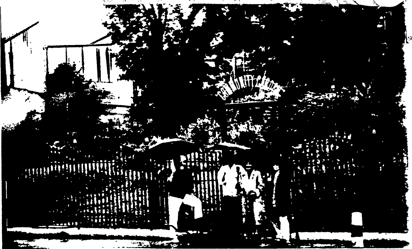
Completed railings and gates: Summer 1988
