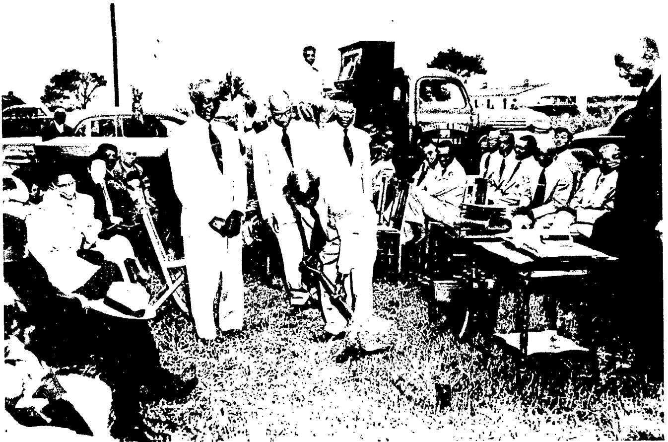
Reverend Walter Weems breaks ground for the new John Wesley AME Church building on Ogden Avenue, 1953. Photograph courtesy of Georgia Robinson and Barry Ballard.
