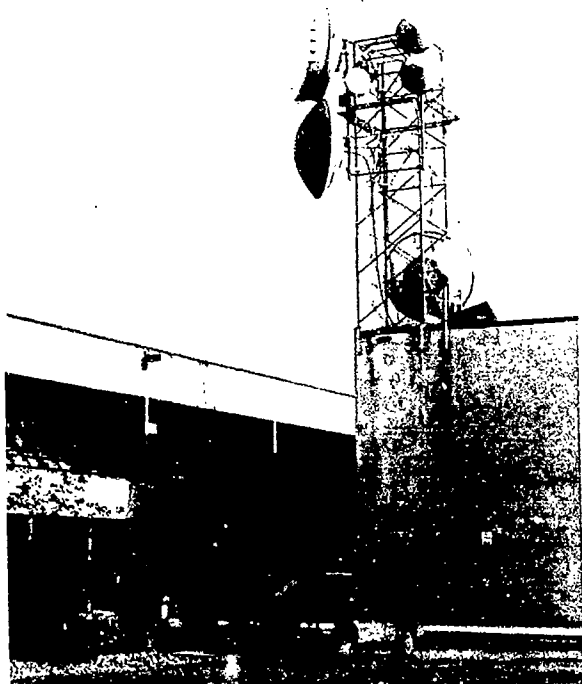
Microwave and satellite dishes at the University of Alaska at Anchorage.
