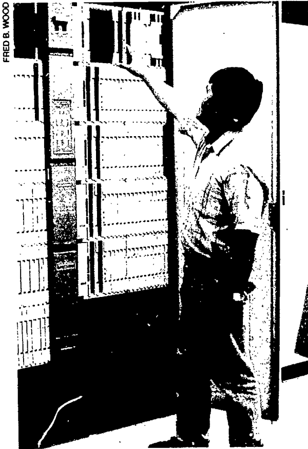
Digital switching center at the OTZ Telephone Cooperative in Kotzebue, Alaska. Rural and urban areas alike depend on modern digital switching and transmission technologies to provide high-quality, low-cost telephone service.
