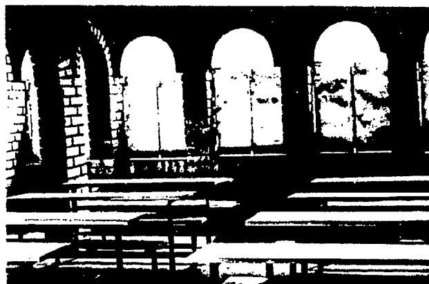
Interior view of a classroom built in Sudan with assistance provided under the "Feasibility Study on the Development of Low-Cost Educational Buildings in Arab LDCs". The prototype utilizes improved local construction techniques, i.e. stabilized soil block walls, corrugated fibre-reinforced roof sheets and stabilized soil tiles laid on compacted earth floors.
