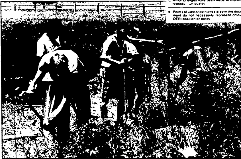
Interagency collaboration is one key to successful employment for persons with disabilities. Here, students from Black Hills Special Services Cooperative (BHSSC) build a fence in a collaborative work project between BHSSC, the U.S. Bureau of Land Management, and Job Service of South Dakota. See story page 6.
