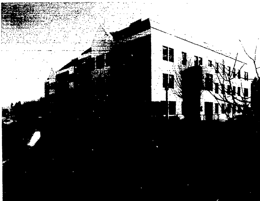
The Boston College Chemistry Building. Entrances at the first floor and lower level are linked inside by a stepped lounge and outside by landscaped terraces.
